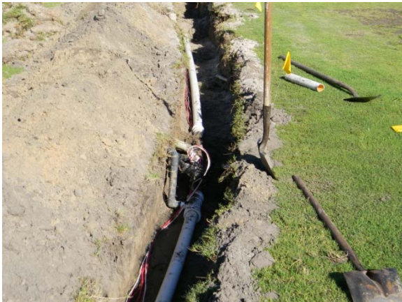
Photo by Randy Doell One of the sprinkler heads being installed.
