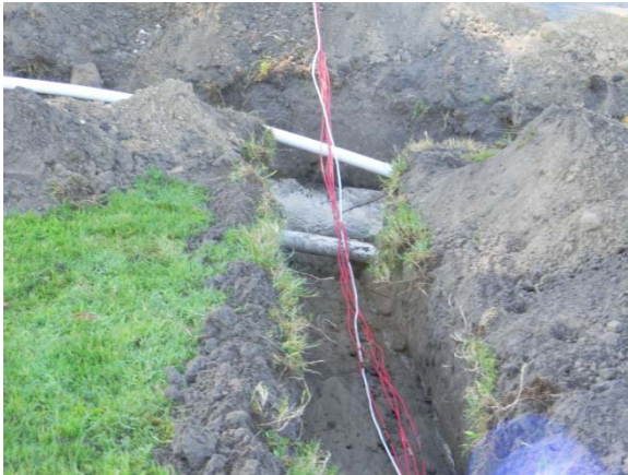
Photo by Randy Doell Wiring being carefully laid
