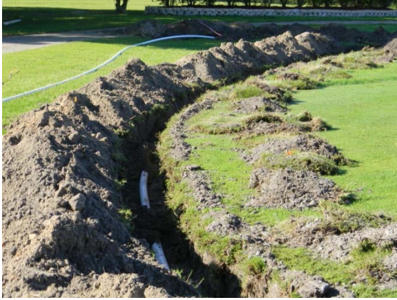
Photo by Randy Doell Pipes, wires and heads being installed
